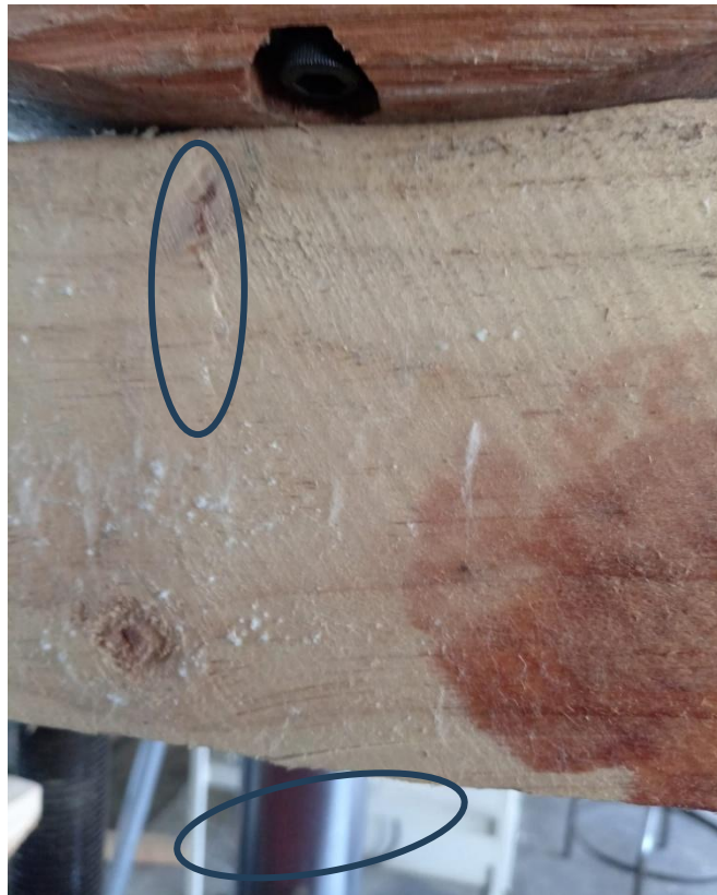
Photo 1: compression and tension failure
